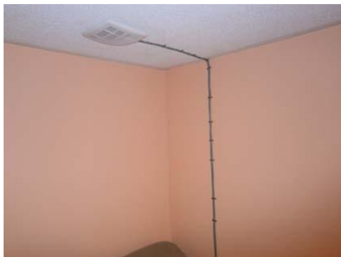
Picture 5 Coaxial Cable Going Into my Basement
