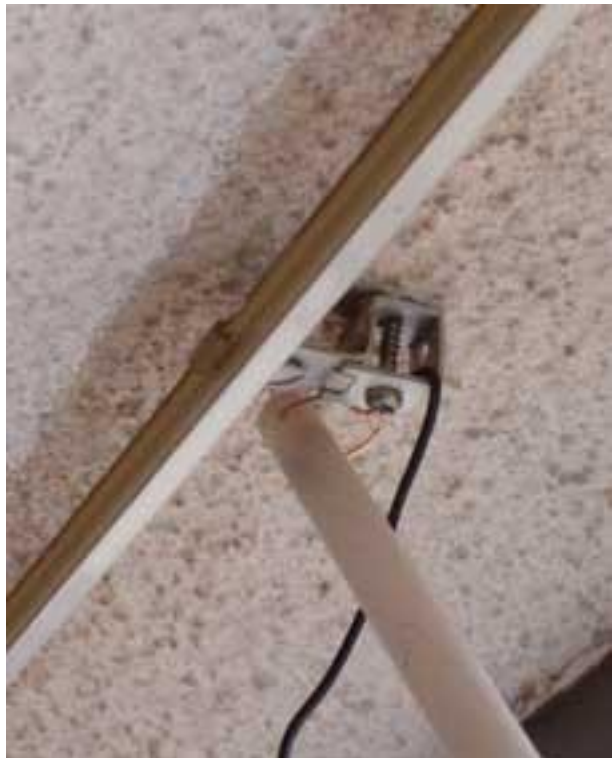
Antenna hung up to eave
