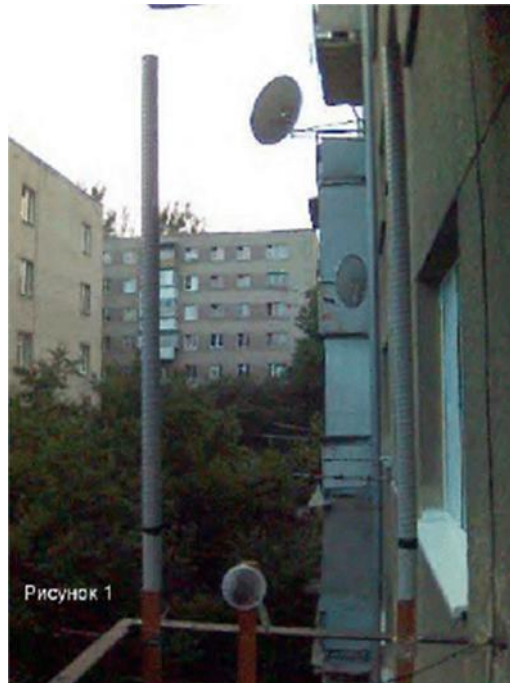
Figure 1 UR5WCA Balcony Helical Antenna
