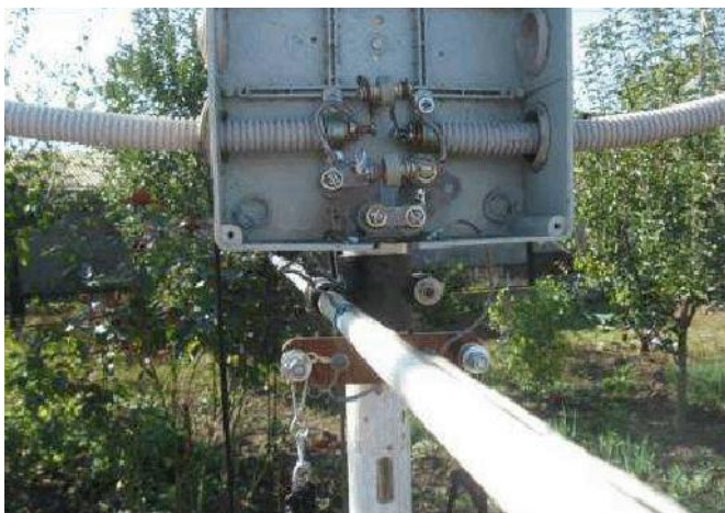
Picture 2 Mounting of the Plastic Tube and Wire Montage of the Horizontal Wires
