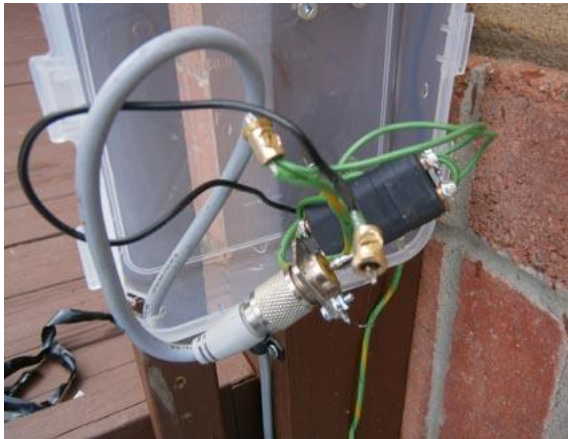
RF Transformer with Insulated Windings at the Beverage Antenna. Open Plastic Food Box
