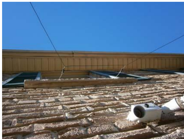
Picture 2 Center of the Simple Broadband Antenna for the 40- meter Band
