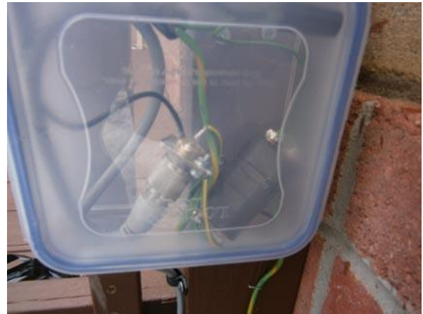
RF Transformer with Insulated Windings at the Beverage Antenna. Closed Plastic Food Box
