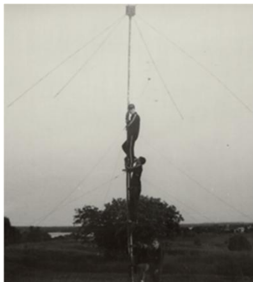
Installation of the Square for 10- 15- 20-meters
