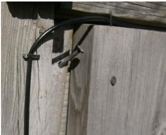
Figure 13 Staped Wire of Beverage Antenna
