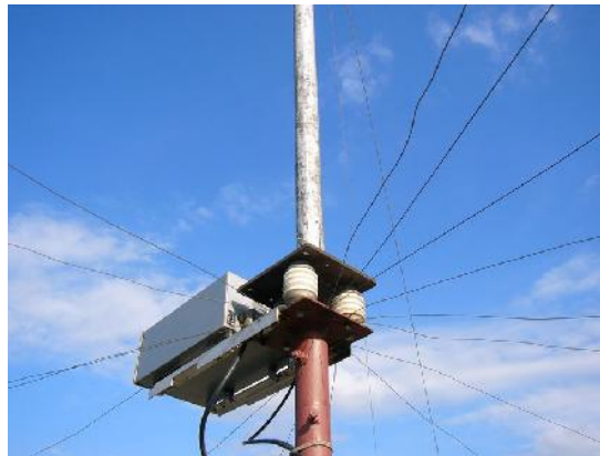
Ground Plane. Box with Matching Circuits
