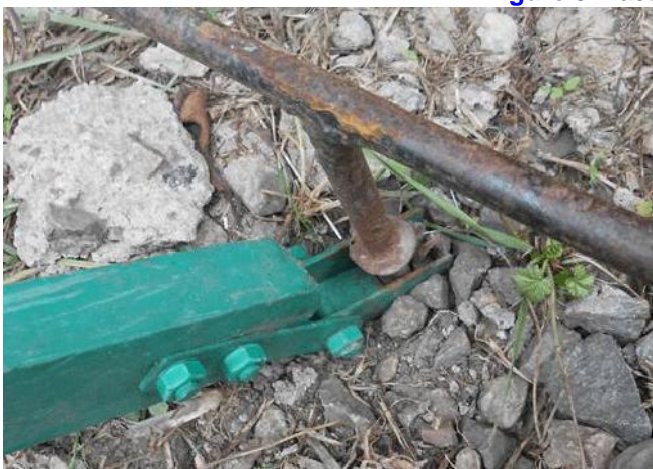
Figure 4 Strut fastened to the ground
