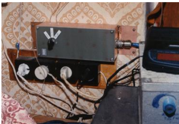
Box with RF Transformers Installed Near a Window
