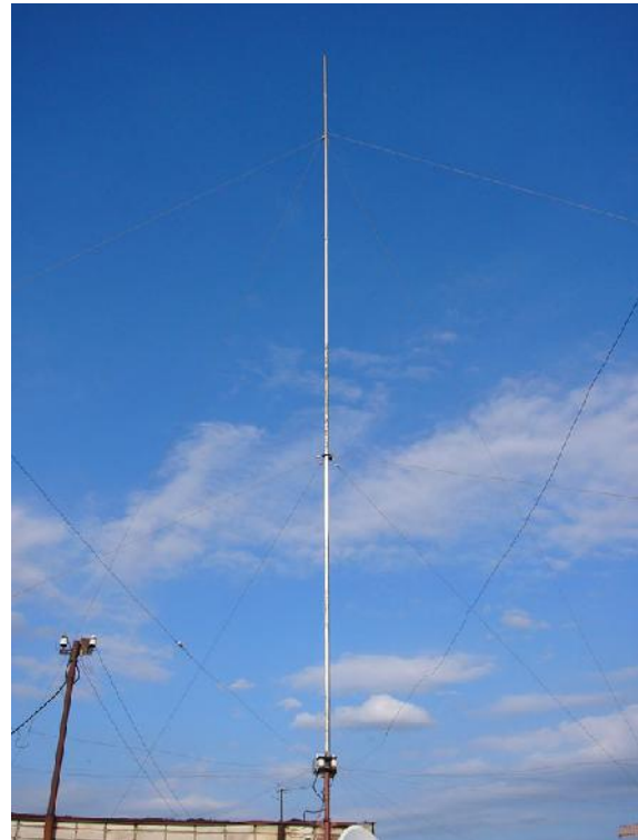
Ground Plane. General view
