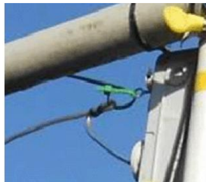
Picture 5 Horizontal Wires at Connection Box
