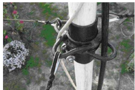
Picture 3 Jointing Mast's Tubes
