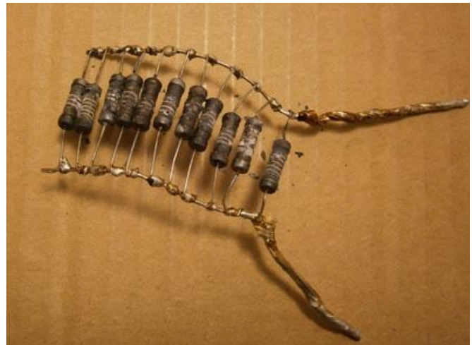
Burned Termination Resistor
