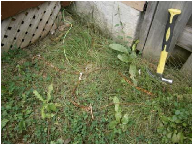
Figure 12 Grounding at the Antenna
